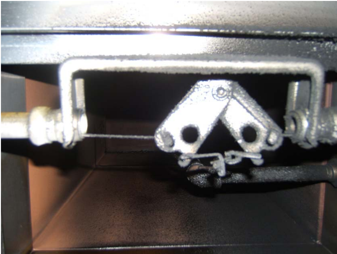
FIRE PROTECTION LINKS AND DUCTS STAY CLEAN AFTER 2 ½ YEARS
