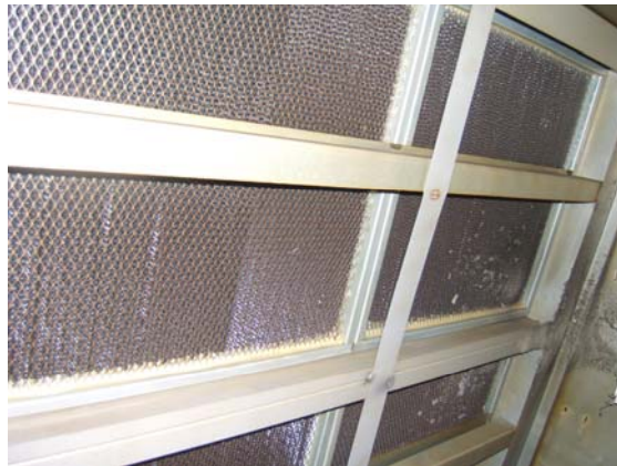
FILTER SECTION INTERIOR
