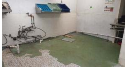
STRIPPED DOWN ROOM
