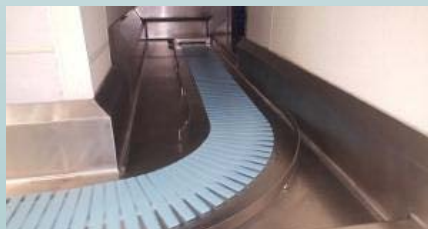
ADDING THE NEW BELT TO DROP OFF WINDOW
