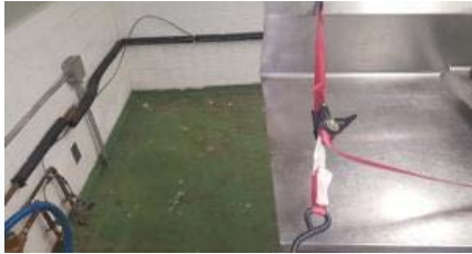
PULLING OLD UNIT FROM WALL
