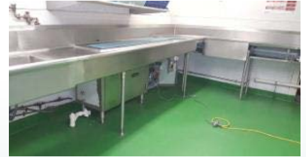
COMPLETED UNIT & CLEAN FLOOR
