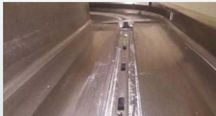
REBEDDING THE TUNNEL
