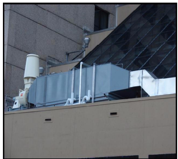
12,000 cfm CAS Rooftop Installation
