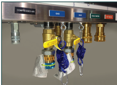
Labeled quick disconnects
