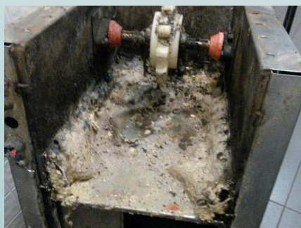
REMOVING OLD RETURN AND WASHER
