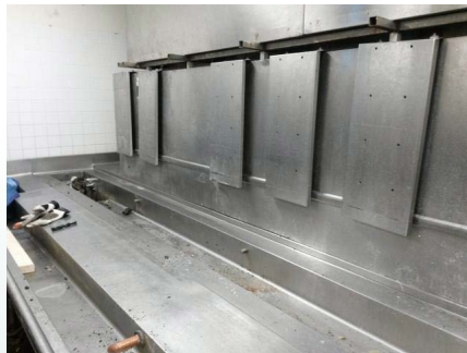
REMOVING OLD KNUCKLE BELT
