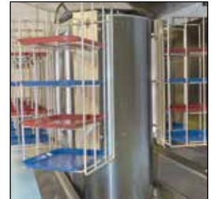
**Vertical Systems** – Complete multi-floor shaft work and cleaning insures uninterrupted delivery of fresh meals along with automatic return of soiled dishes. Multiple trays can be loaded or unloaded from both sides of the shaft for maximum efficiency.
